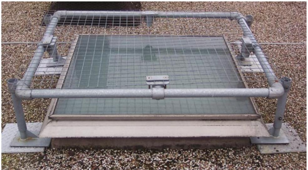
*Covers can be fitted to existing roofs or included as part of the design
