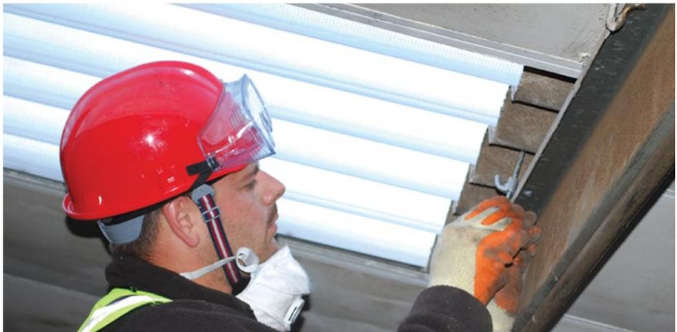
*Securing fixings to newly installed sheet*
