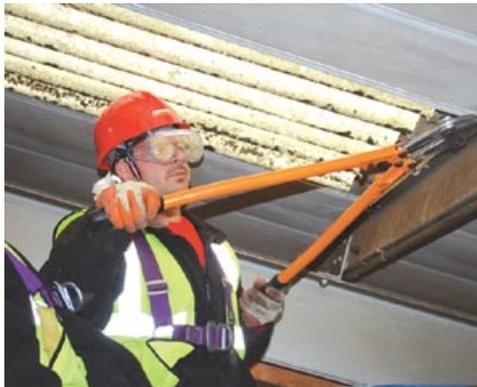
*Removing hook bolts from existing sheet*
